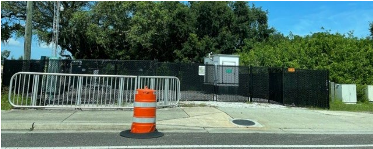
Figure 3 | County Lift Station (2021 HDR Site Reconnaissance)
