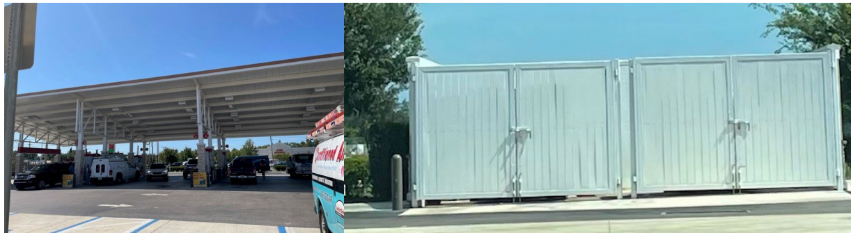
Figure 4 | WAWA (2021 HDR Site Reconnaissance)
